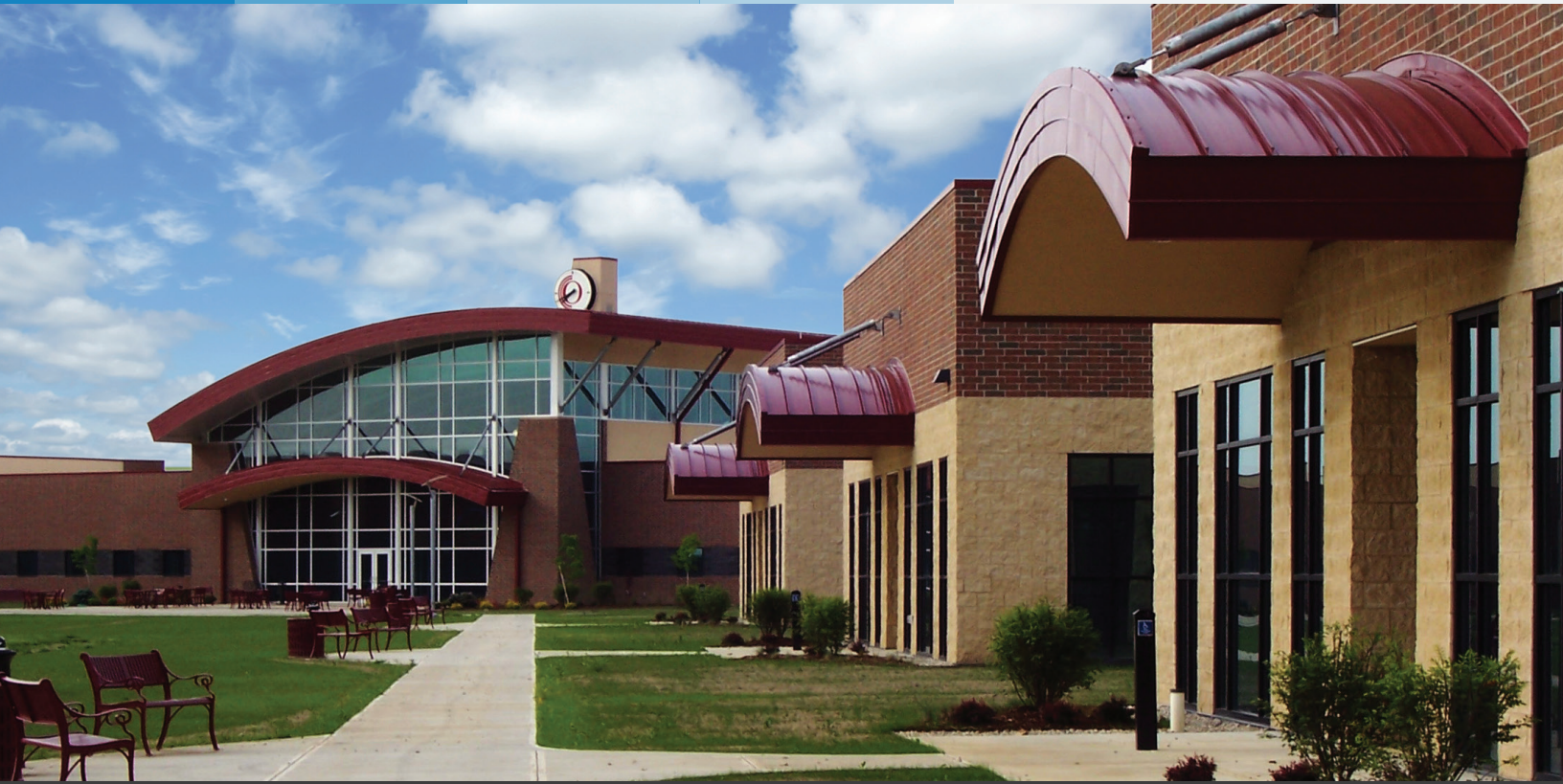
PROJECT: Owens Community College LOCATION: Fredericktown, OH PANEL PROFILE: Curved BattenLok® COLOR: Colonial Red
