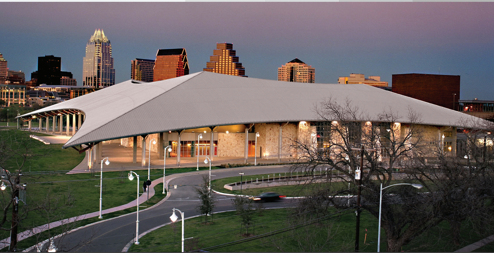
PROJECT: Lester E. Palmer Events Center LOCATION: Austin, TX PANEL PROFILE: SuperLok® COLOR: Galvalume Plus®
