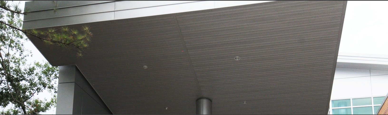
PROJECT: Texaco Service Station LOCATION: Beaumont, TX PANEL PROFILE: QwikLok™ COLOR: White
