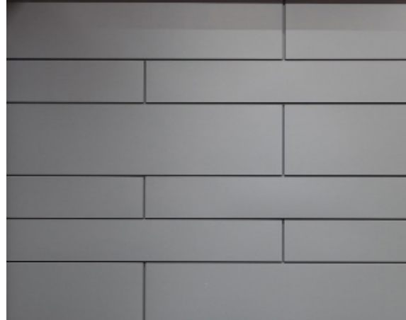
OFFSET HORIZONTAL INSTALLATION
