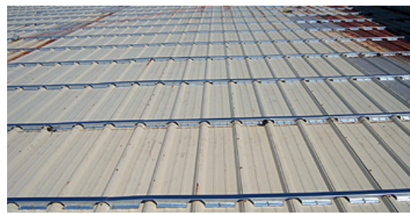
Roof Hugger over existing R Panel
