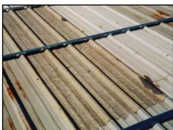
Cut out and trim opening if new skylights are to be installed above, or leave panel in position if skylights are to be eliminated.
