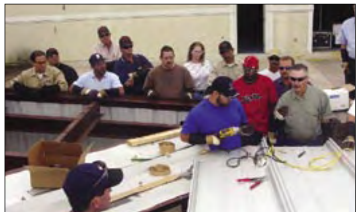
Hands on training for the people that will actually install the roof provides valuable knowledge that otherwise may take years to acquire.
