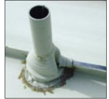
It is almost impossible to seal a rubber roof jack to a panel seam
