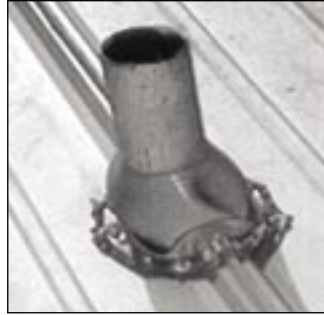
It is almost impossible to seal a rubber roof jack to a panel seam
