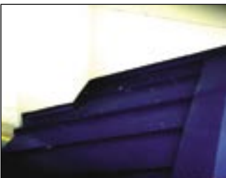
Without a welded aluminum cricket, this offset will probably not perform long-term.
