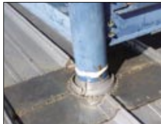
Two-piece pipe curb and retrofit rubber roof jack.
