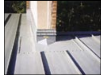
This cricket provides a complete seal at the end of the parapet wall, eliminating the need for surface applied sealant.
